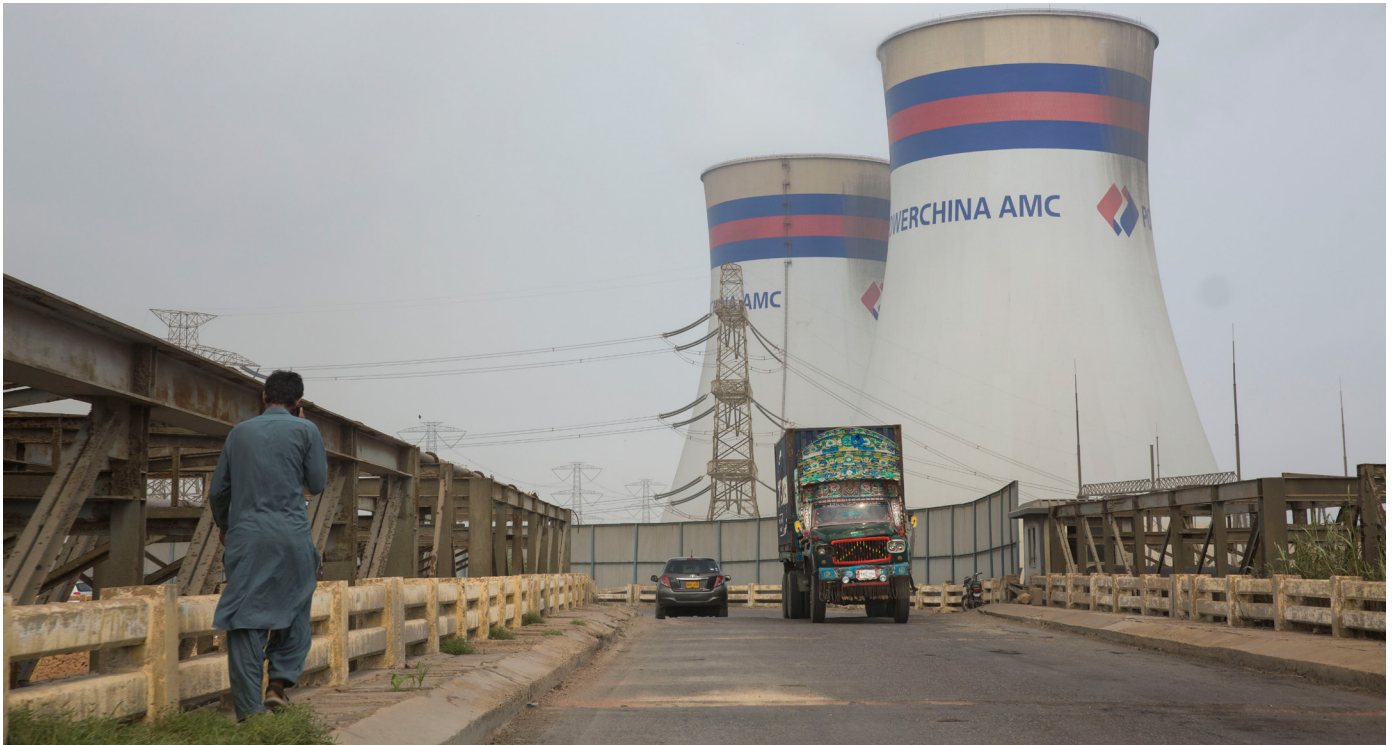
CPEC coal-fired power plant at Port Qasim.
