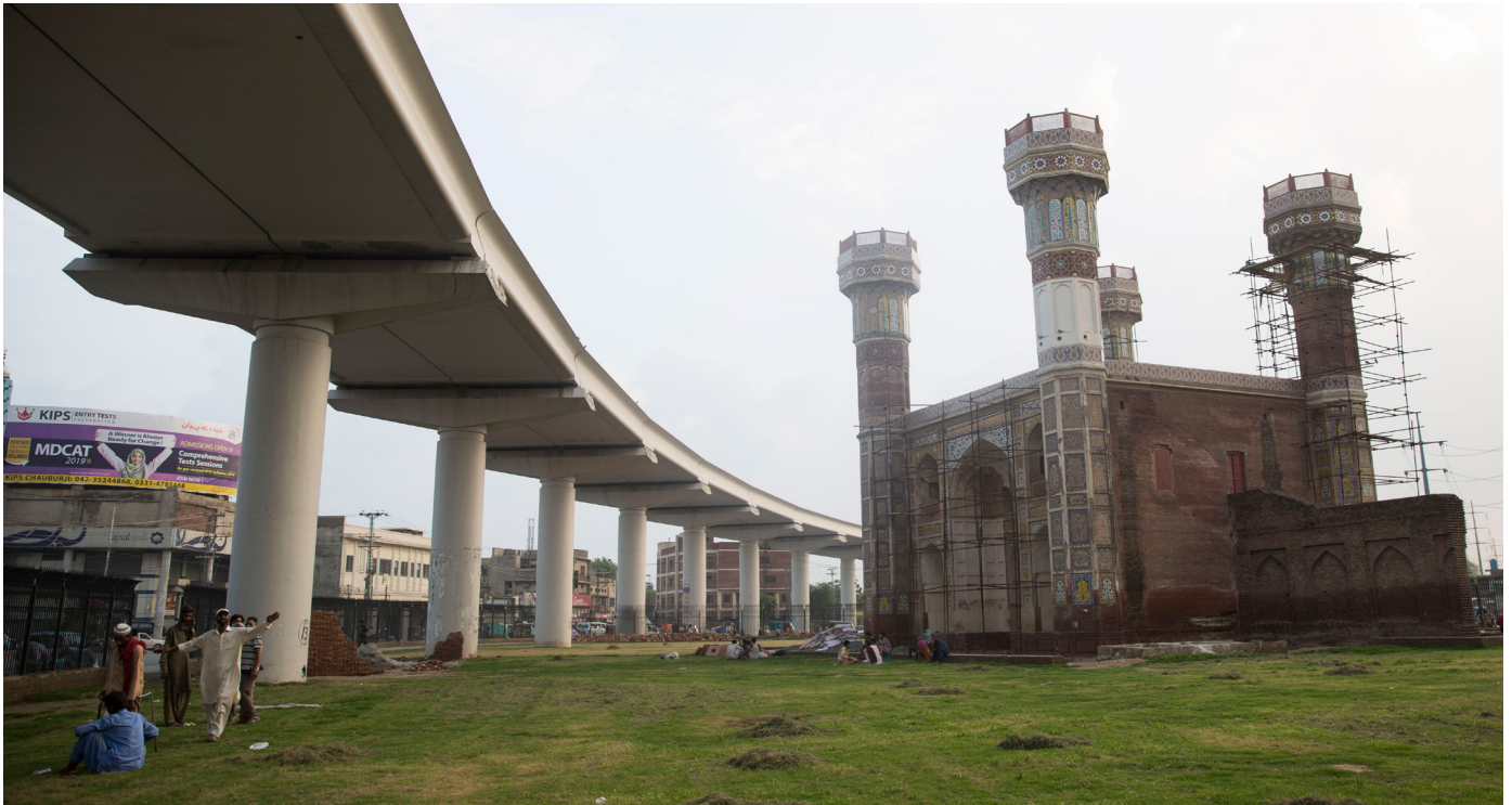
CPEC's Orange Line metro project, Lahore.
