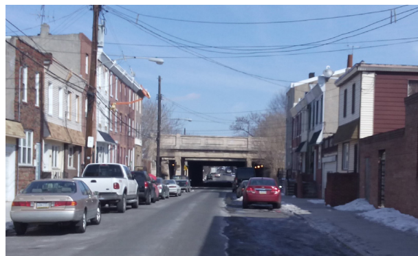
Figure 5: View of the Lehigh Viaduct from surrounding neighborhoods
